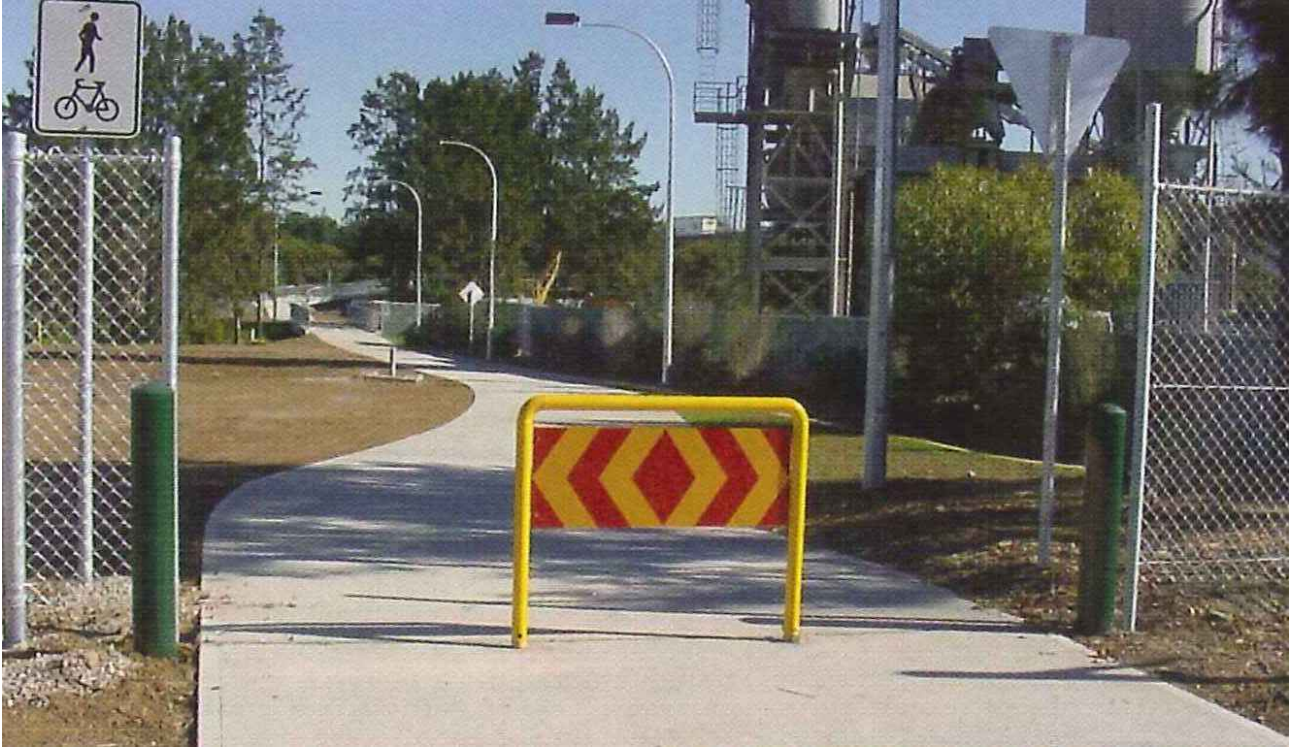
Figure 7.9: Example of U-rail and hazard board treatment
