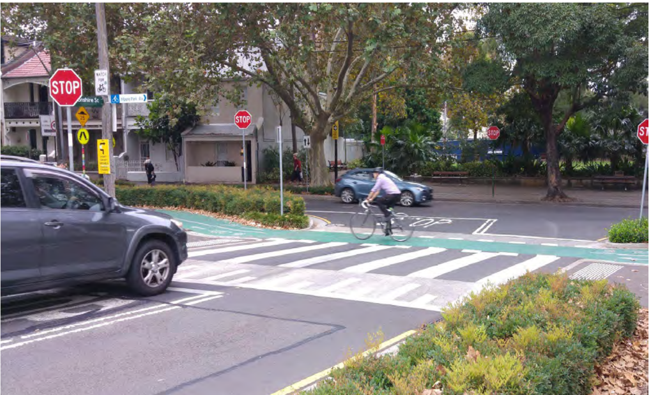
Figure 7.3: Example of an intersection where a path crossing has priority over a side street
