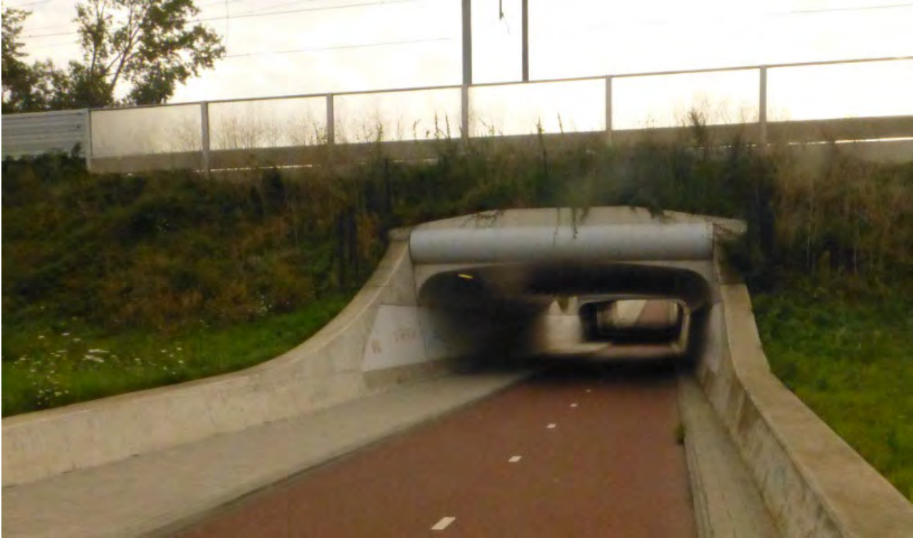
Figure 8.3: Example of a pedestrian/bicycle path underpass
