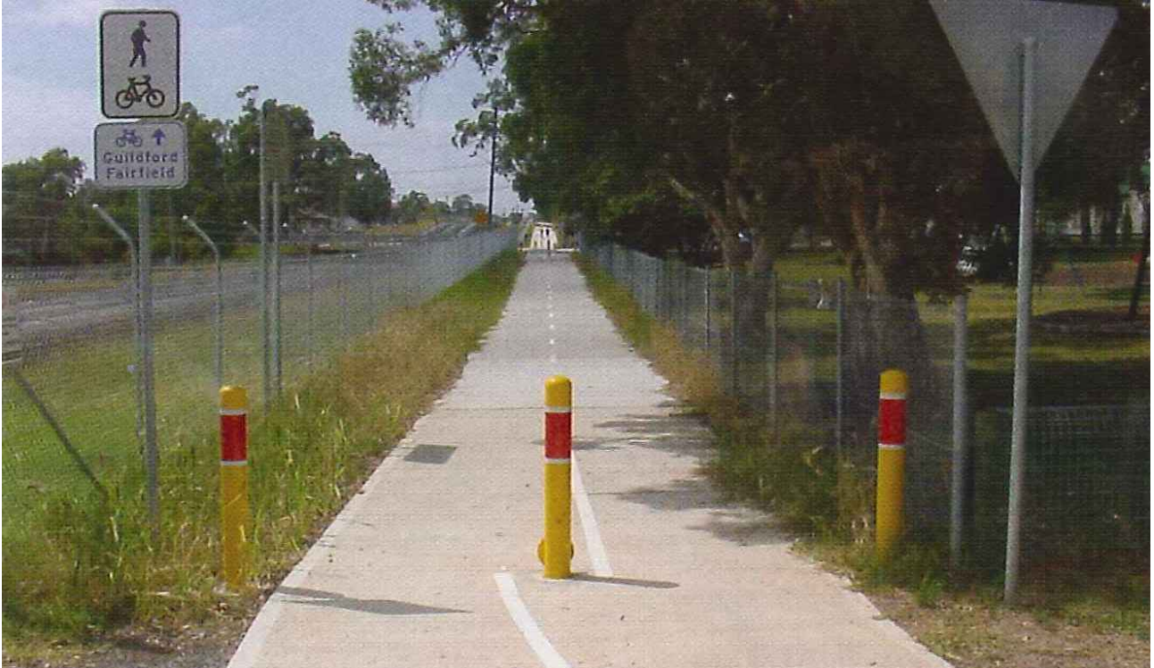
Figure 7.7: Example of a bollard treatment
