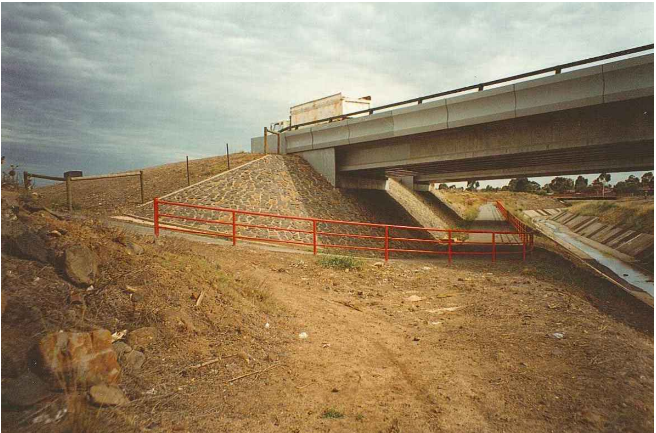
Figure 8.2: Shared path under a bridge abutment
