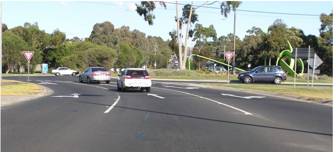
Figure 7.1: Example of a landscape treatment in the central island of a large roundabout
