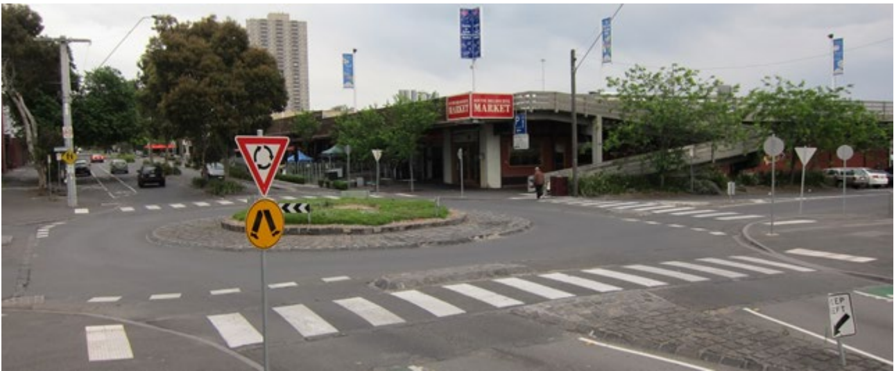
Figure 5.1: Local road roundabout with wombat crossings on all intersection arms along the pedestrian desire line (Cecil Street, South Melbourne)
